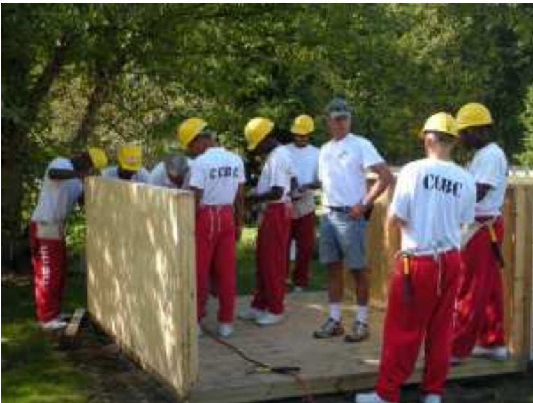
Tom & Carl supervise the crew reassembling the shed
